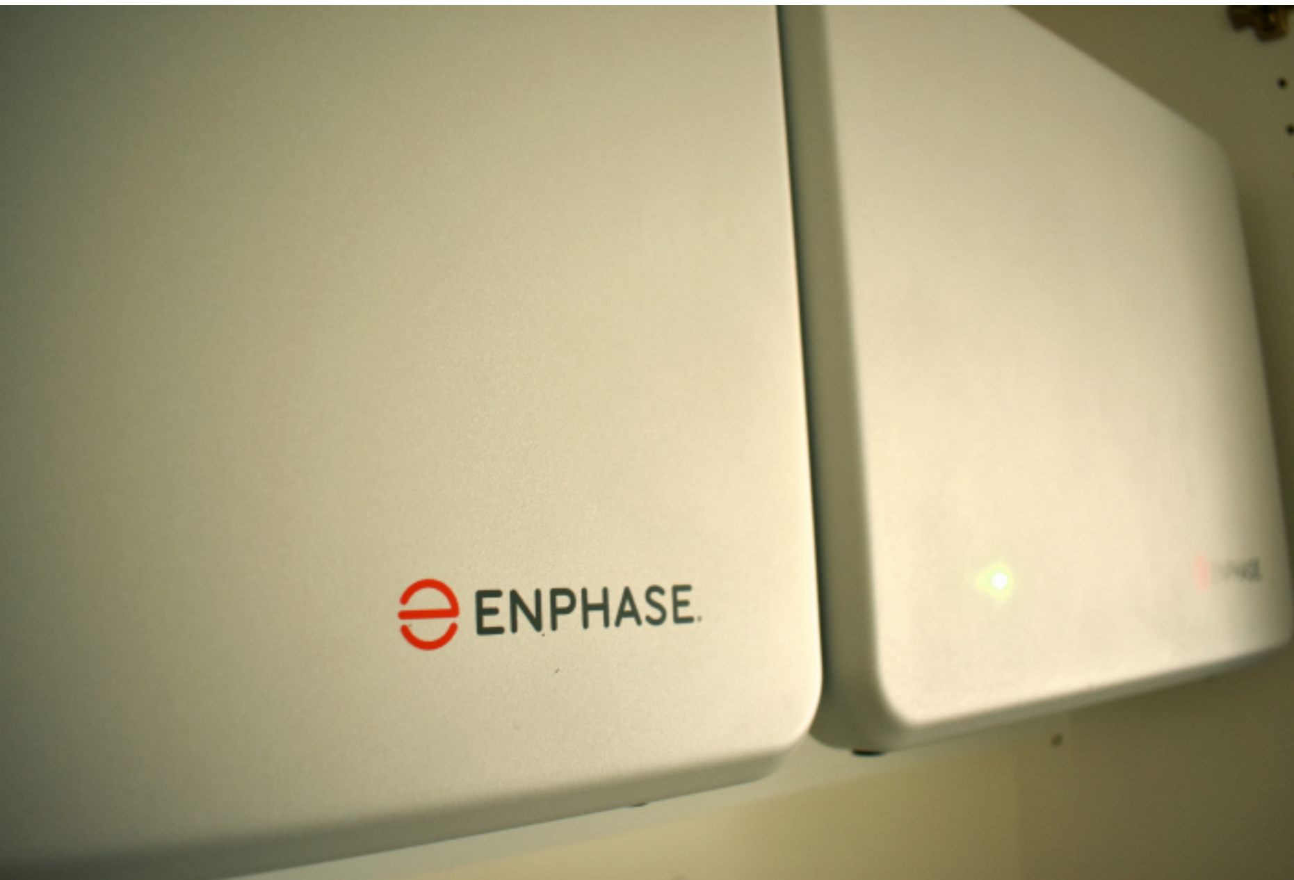
A series of four Enphase batteries installed in a Green Efficient Living customer's home.
