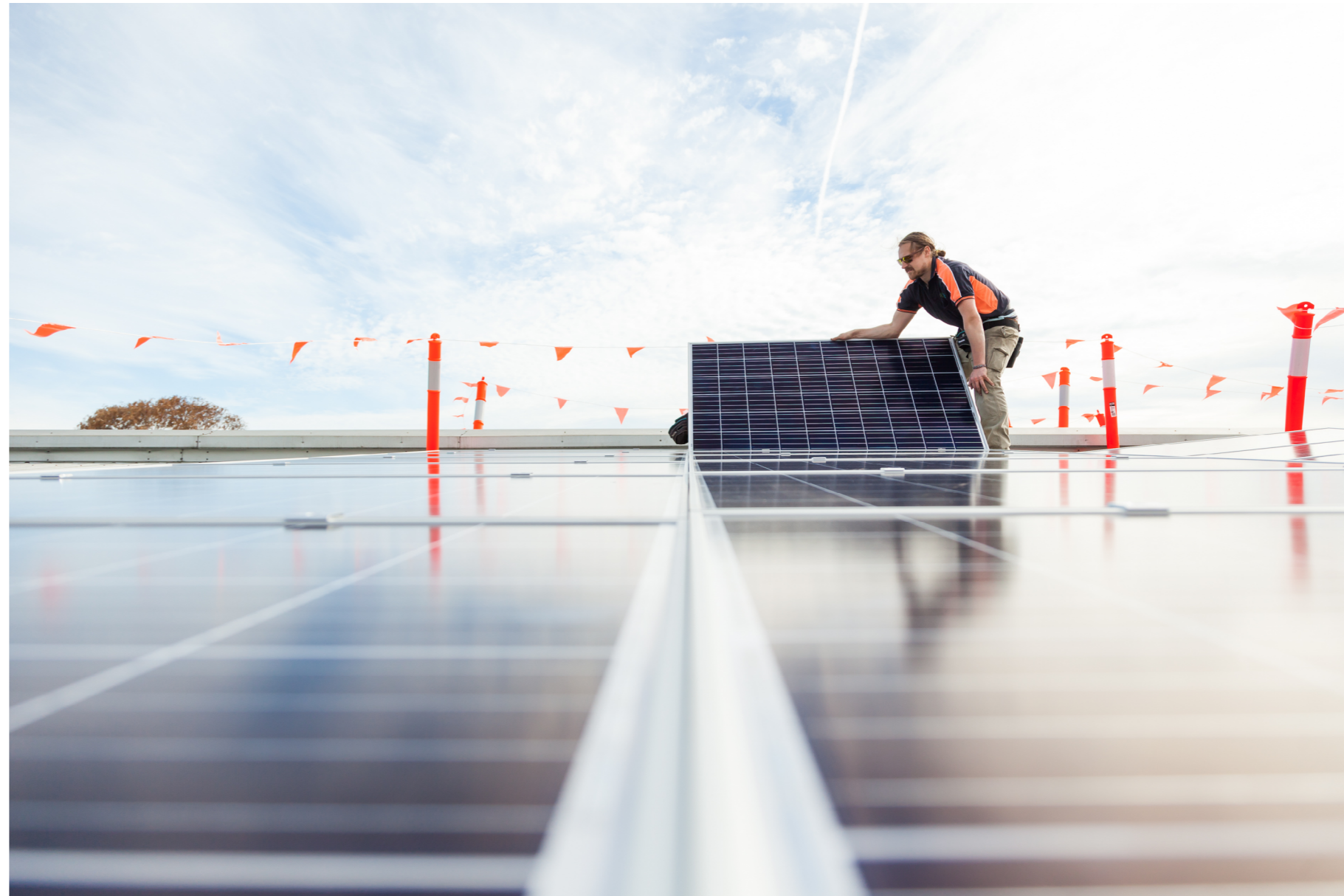
Green Efficient Living installing a commercial solar system.
