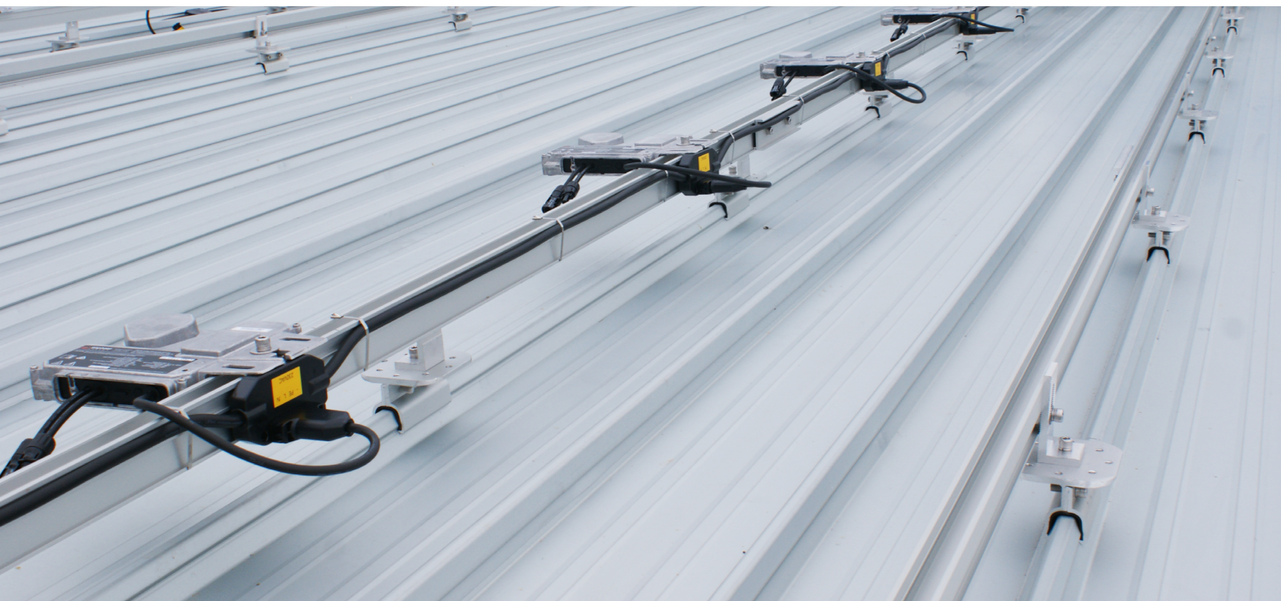
One of Green Efficient Living's installations demonstrating what your system is meant to look like beneath the panels with no loose or sagging wiring.
